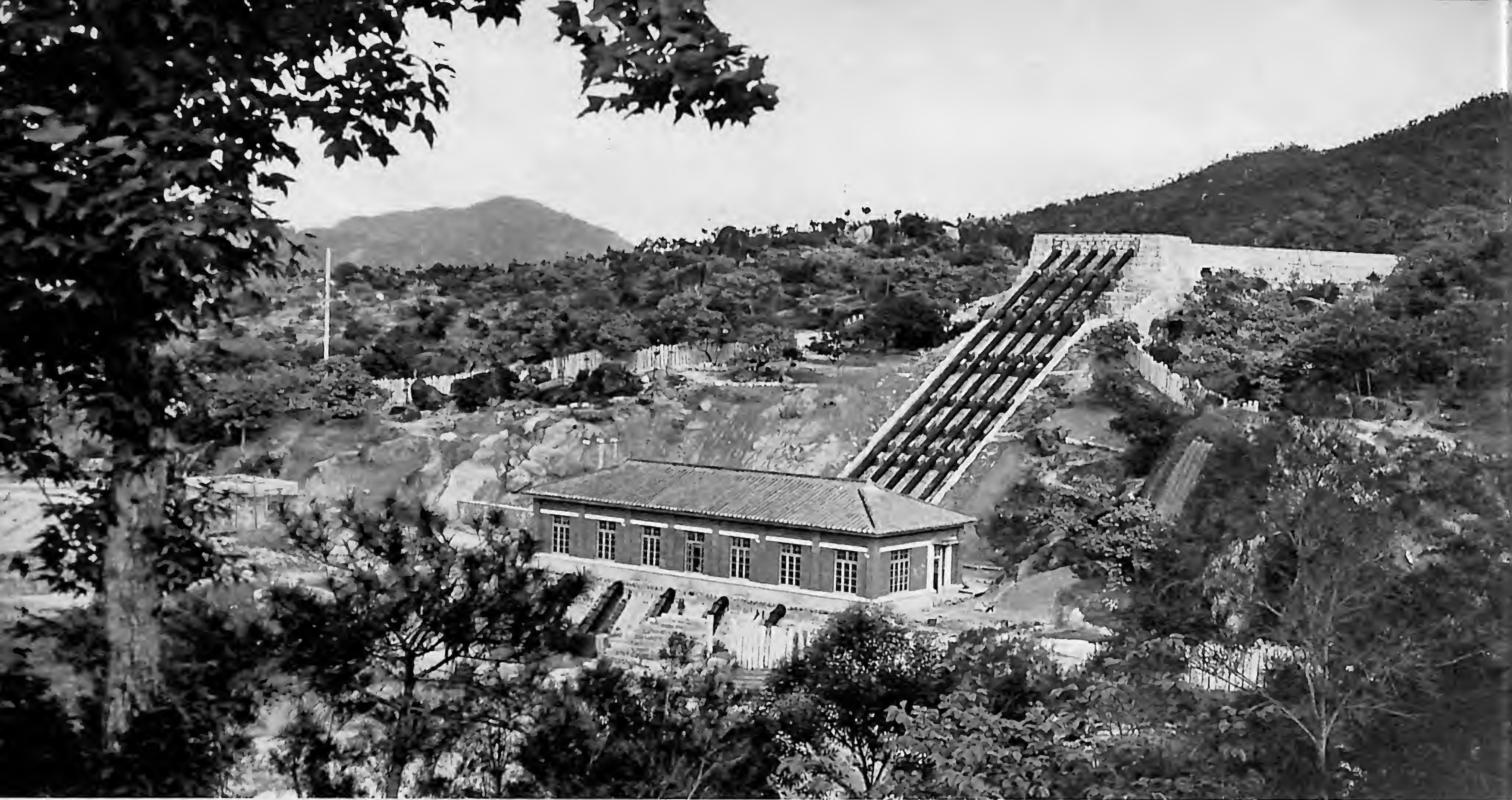
The Shihtso Electric Pumping Station on the Hsi River. It can raise water 28 metres.
